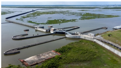
Figure 1. “Protection”: sea wall, Louisiana built after Hurricane Katrina .
