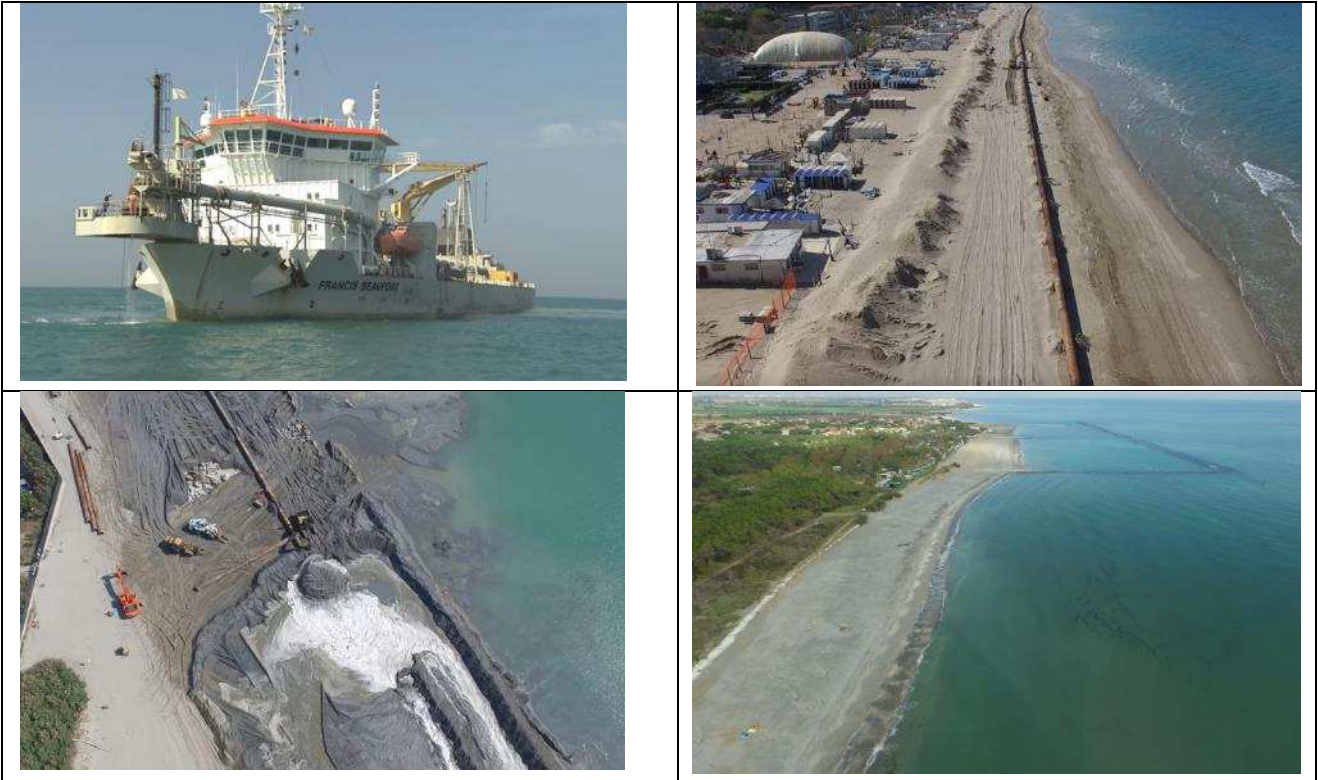
Figure 5- Nourishment intervention of 2016: the trailing suction hopper dredge (top left), the pipeline(top right), a nourishmentyard (bottom left), the beach of Lido di Dante after the nourishment (bottom right).
